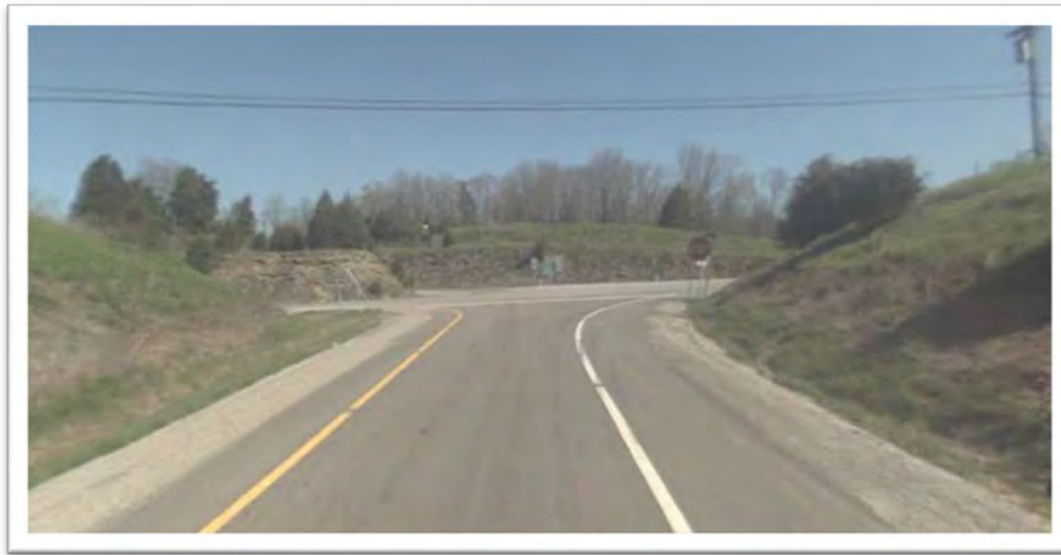
Figure 20 – On the ramp from northbound I-75 looking north to KY 36
