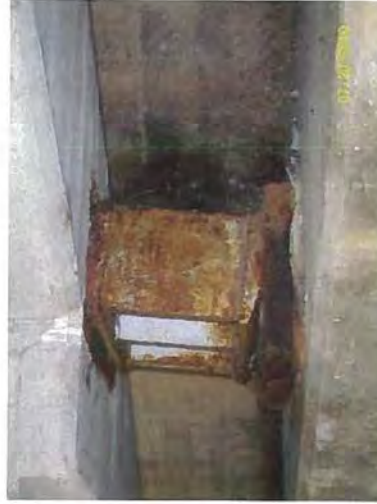
Rocker # 2 at the forward abutment
