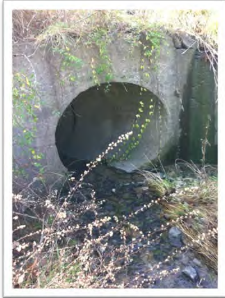
Figure 2 - 52" Pipe North of KY 36, inlet
