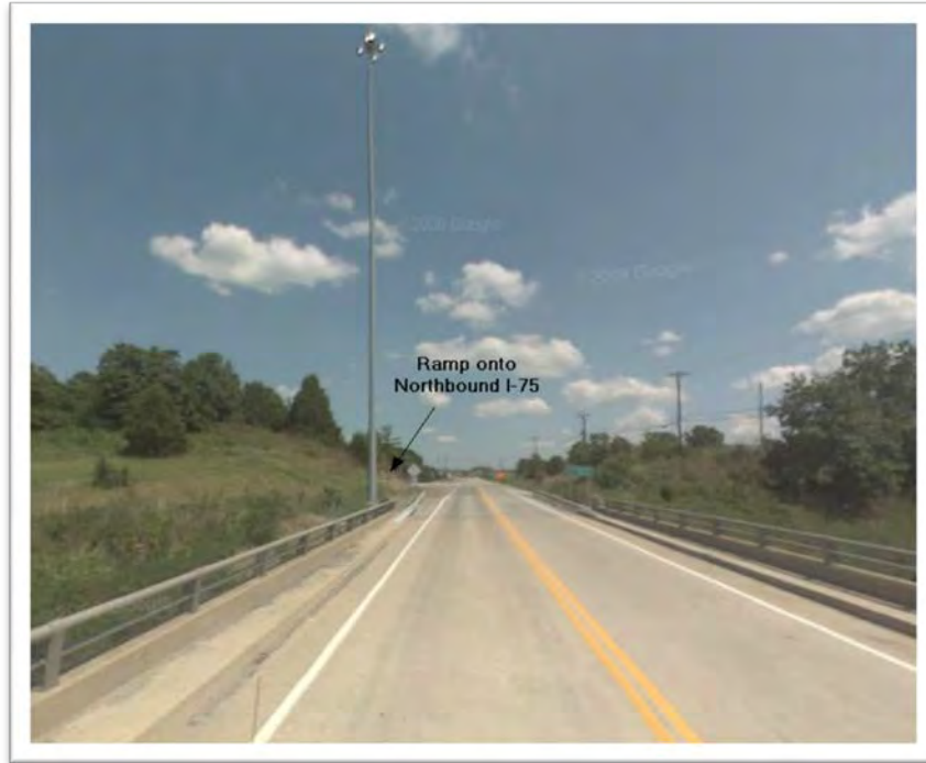
Figure 18 – On the KY 36 Bridge over I-75, looking east to the ramp onto northbound I-75
