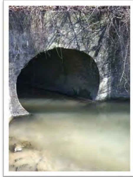
Figure 3 - 52" Pipe South of KY 36, outlet
