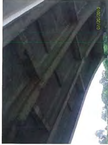
Bottom side of span # 2 over KY-75 Southbound
